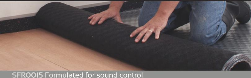
SFR Sound Insulation is a flat, resilient underlayment used directly under all floor finishes, yielding exceptional results even under hard surface flooring and over concrete and wood joist construction.
